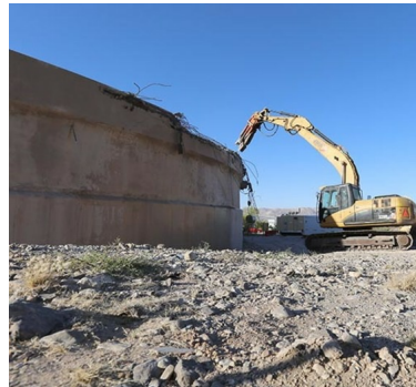
Jackson Reservoir demolition
